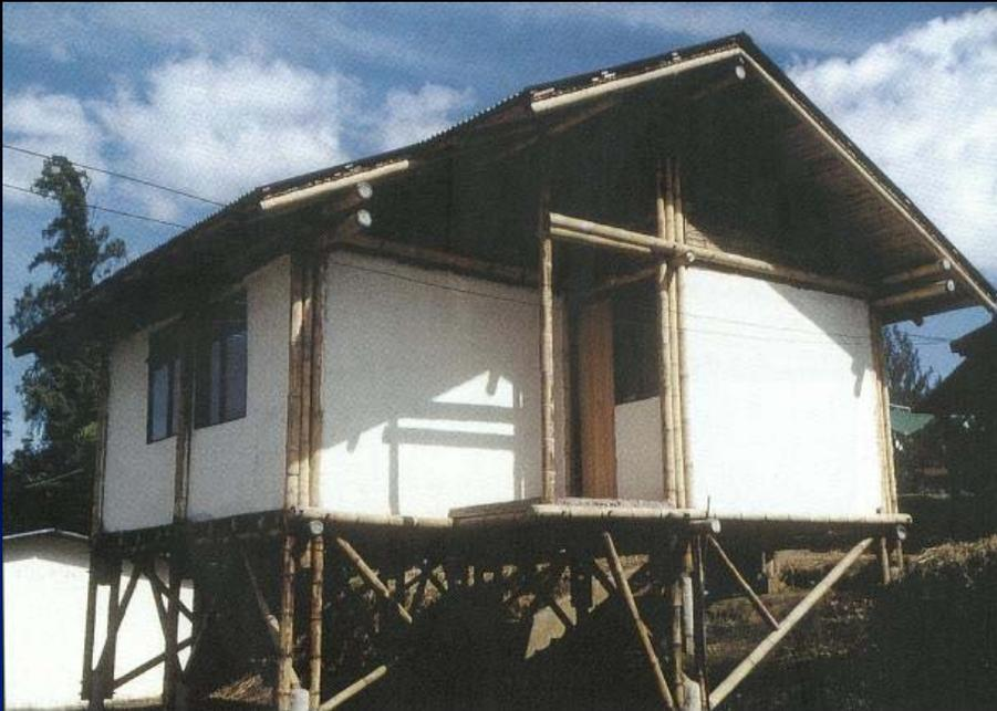
Fig. 103: *Prototype of a bamboo house with elevated floor (Costa Rica)*
