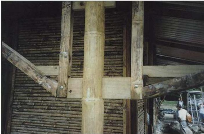
Fig. 74: Connection between truss and column
