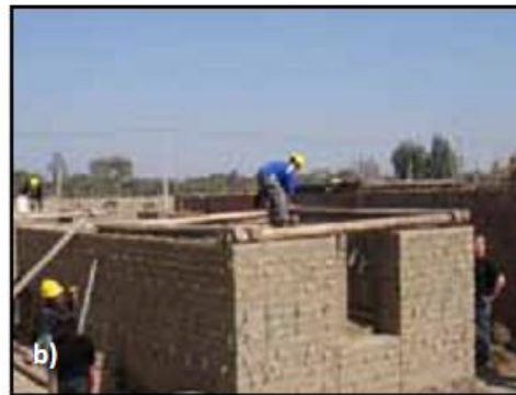
Figure 4.1 Ring beams made of different materials: a) Wood, b) Eucalyptus logs, and c) Bamboo
