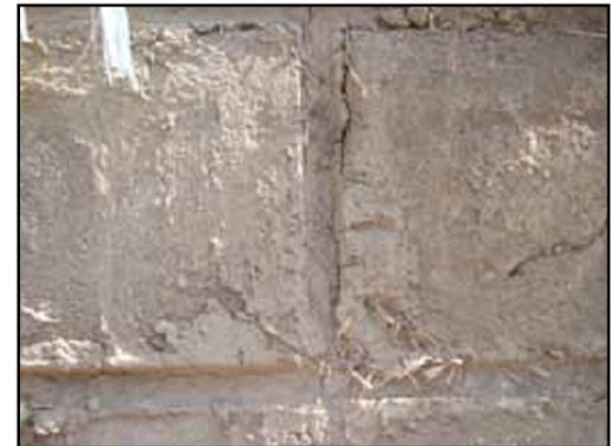
Figure 3.8 Mortar joins that are uniform and completely filled
