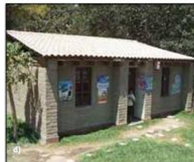
Figure 4.3 Construction with cane reinforcement in Peru and El Salvador: a) Placement of cane reinforcement, b) Vertical and horizontal reinforcement, c) Barbed wire as horizontal reinforcement, and d) House reinforced with cane and pilasters
