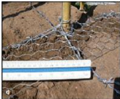
Figure 4.3 Construction with cane reinforcement in Peru and El Salvador: a) Placement of cane reinforcement, b) Vertical and horizontal reinforcement, c) Barbed wire as horizontal reinforcement, and d) House reinforced with cane and pilasters
